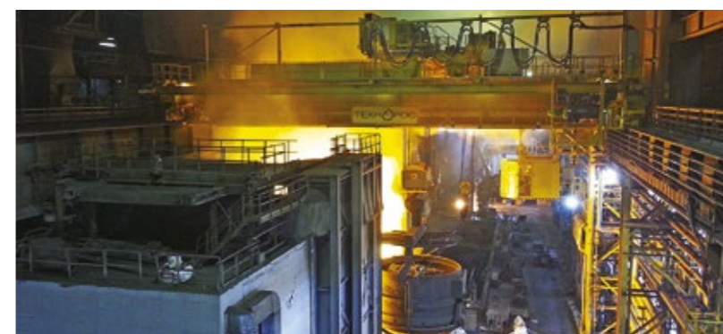
METALLURGICAL BRIDGE CRANES 120+32 / 10-24,5-A8, Y2 Customer: "Belarus metallurgical factory"
